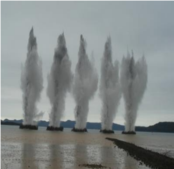
Figure 2. The underwater explosion to open a stream in Spratly Islands 1991 (Le, 1991)
