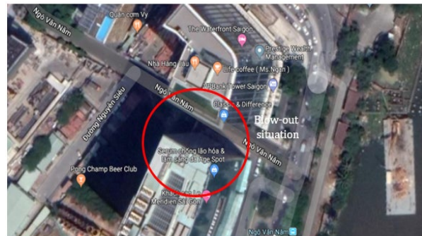
Figure 9. Blow-out at the chainage Km1+500 of the West Line in Hochiminh Metroline No.1.
